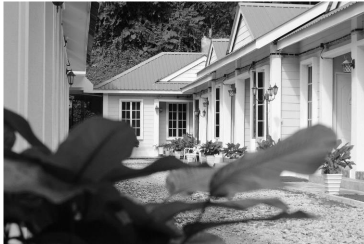
Figure 1: Residential Units in MIMNI
